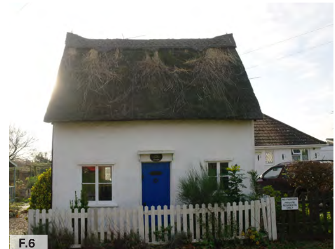
Figure 06: Glen Cottage, Grade II Listed Building.
