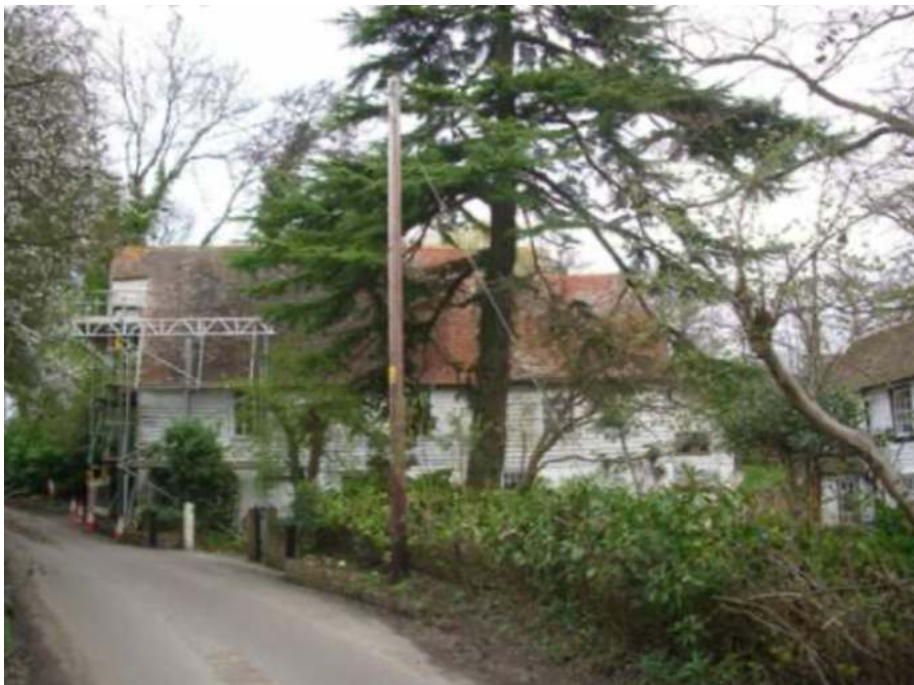
Fig. 20. The Grade II* listed Spring Valley Mill
