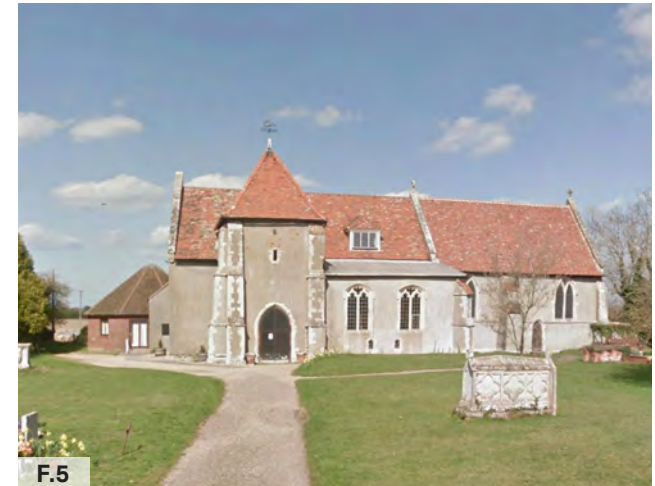
Figure 05: The Church of St Anne and St Lawrence, Grade I Listed Building.
